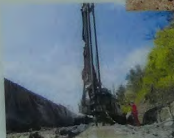
A drilling rig installing the underground barrier of bentonite/cement soil mix.
