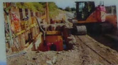
A drilling rig installing the underground barrier of bentonite/cement soil mix.
